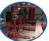
Fire water tank and pumping systems skid
